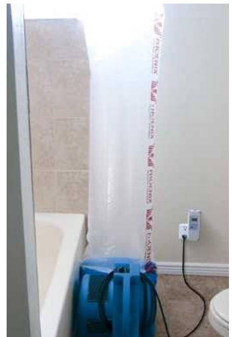
Air mover with ducting controlled by MB230 Exhaust Controller
